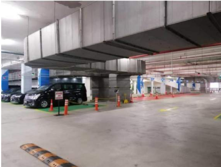
KOMTAR JBCC LEVEL 3 – EXIT TO CAR PARK
